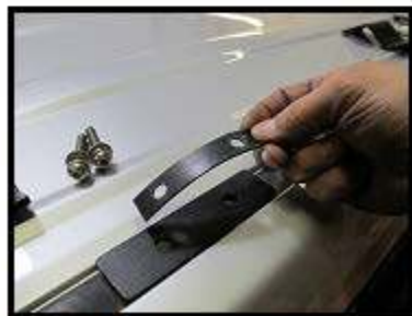
Fig. 13 Place black cover plate over gasket and another gasket on top
