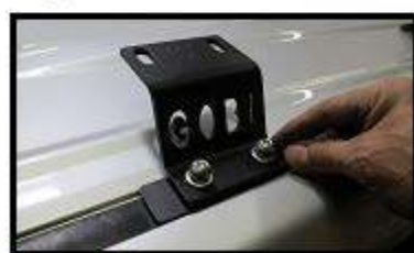
Fig. 15 Install M8x50 screws, lock washers and water proof washer Bag#3 and snug down. Apply the same procedure to the other 5 brackets.
