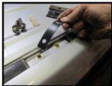
Fig. 10 Place gasket on roof top around mounting holes.
